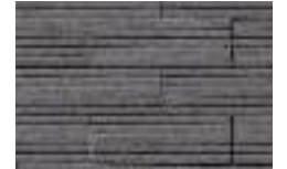
BK-1106 without grouting
