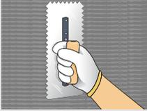
Apply a generous layer of mortar adhesive across the wall using the notched edge of a trowel, creating a "combed" surface pattern.
